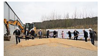
Official ground-breaking ceremony for the construction of a new production hall by District Administrator Willibald Gailler, Berching's Deputy Mayor Christian Meissner and HUBER's Executive and Supervisory Boards
