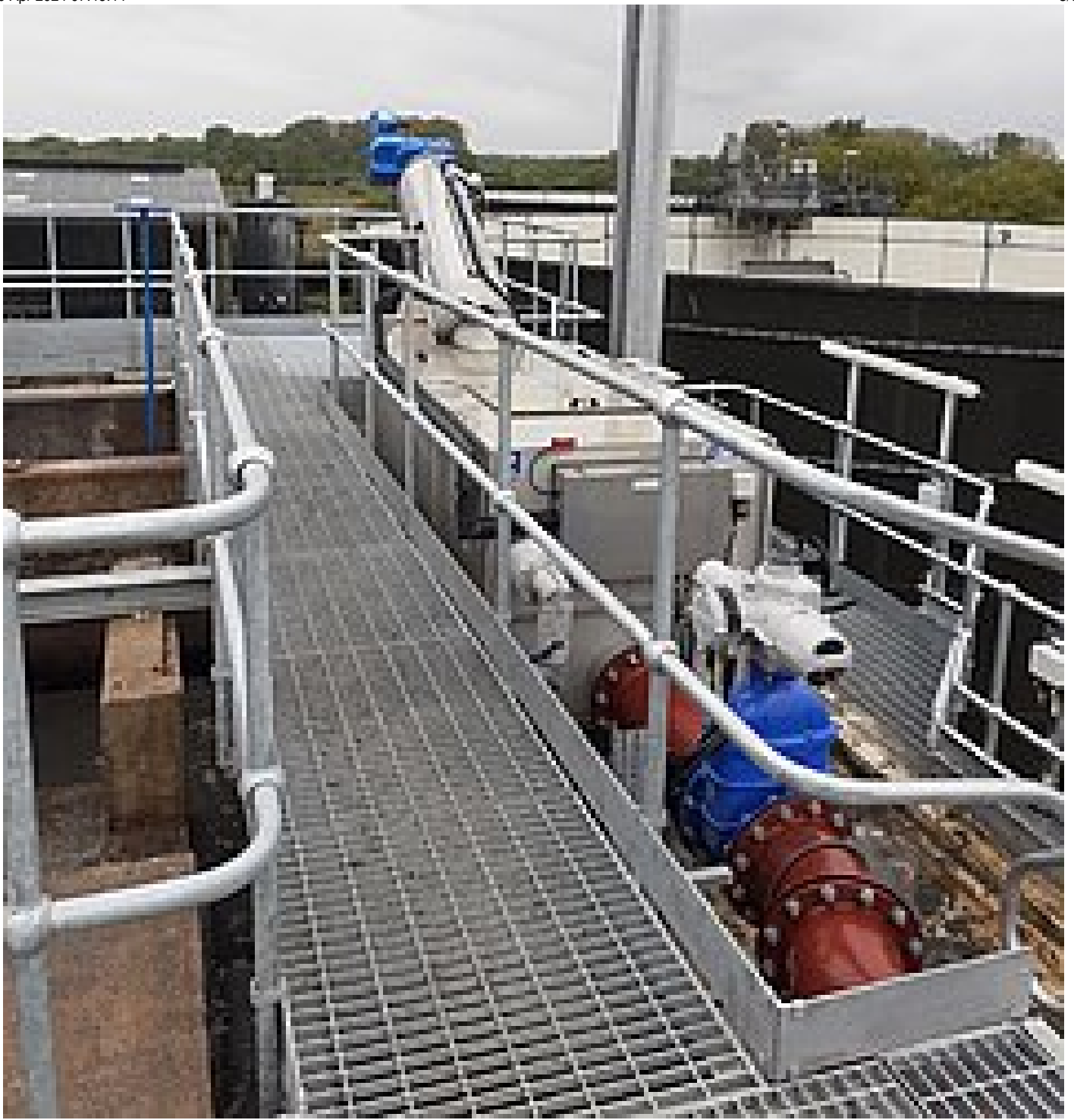
New screen adjacent to the old channel
