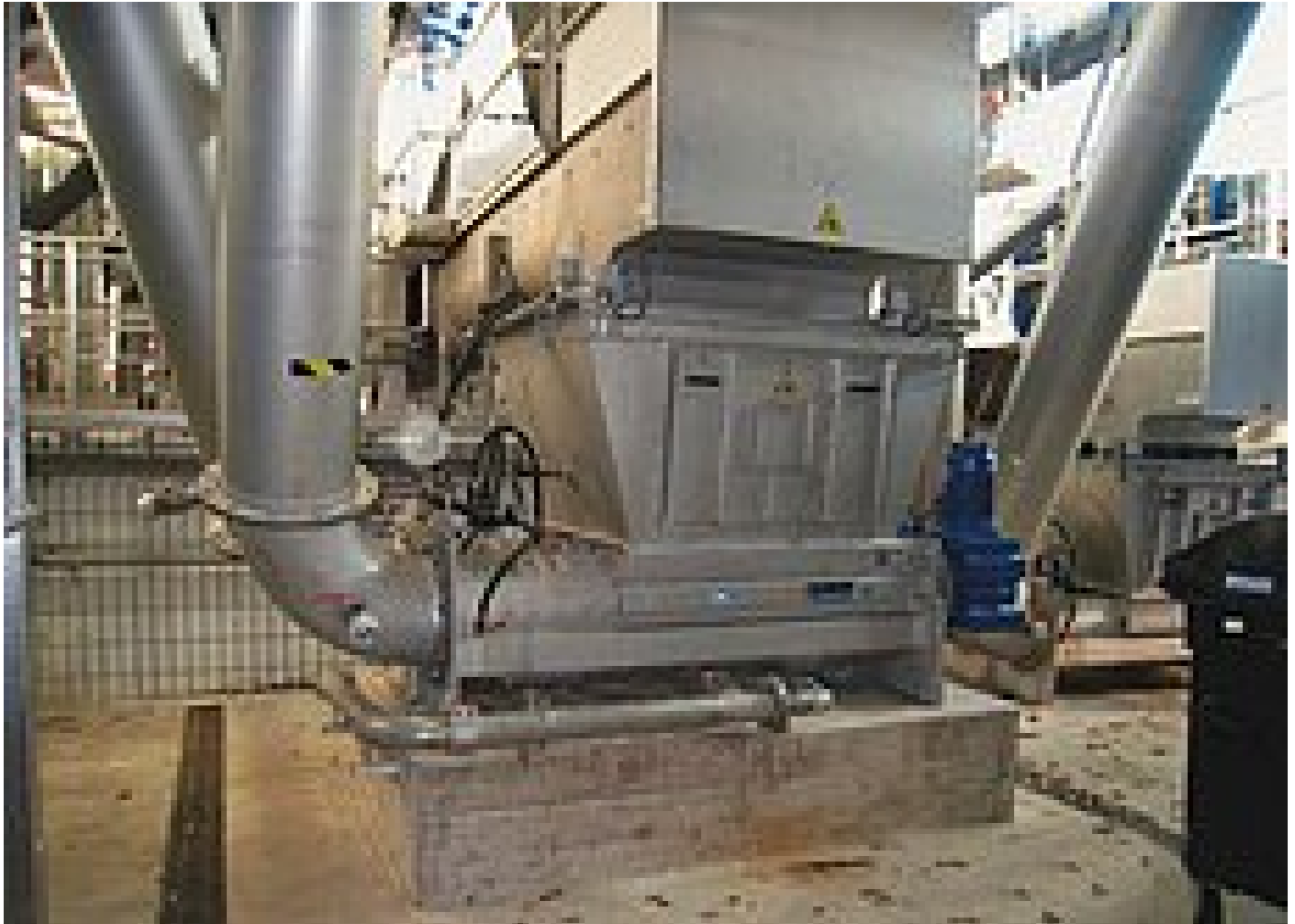
HUBER Wash Press WAP® 2x8 with 16m 3 /h throughput each
