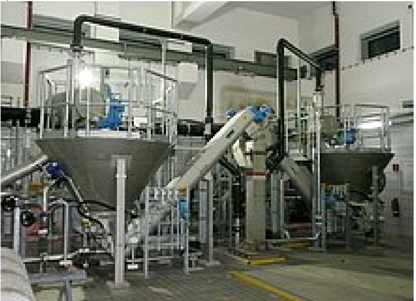
In operation since 2011 – HUBER COANDA Grit Washer units, type RoSF 4, size 16 l/s
