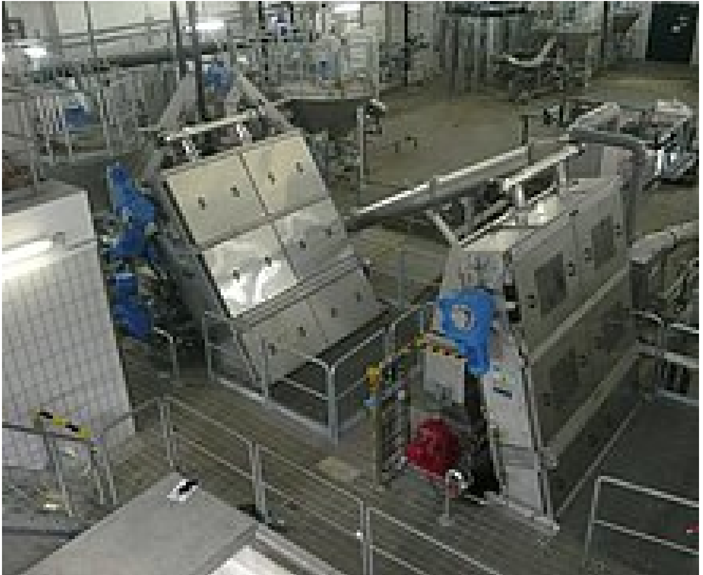
Line 1 shortly after start-up
