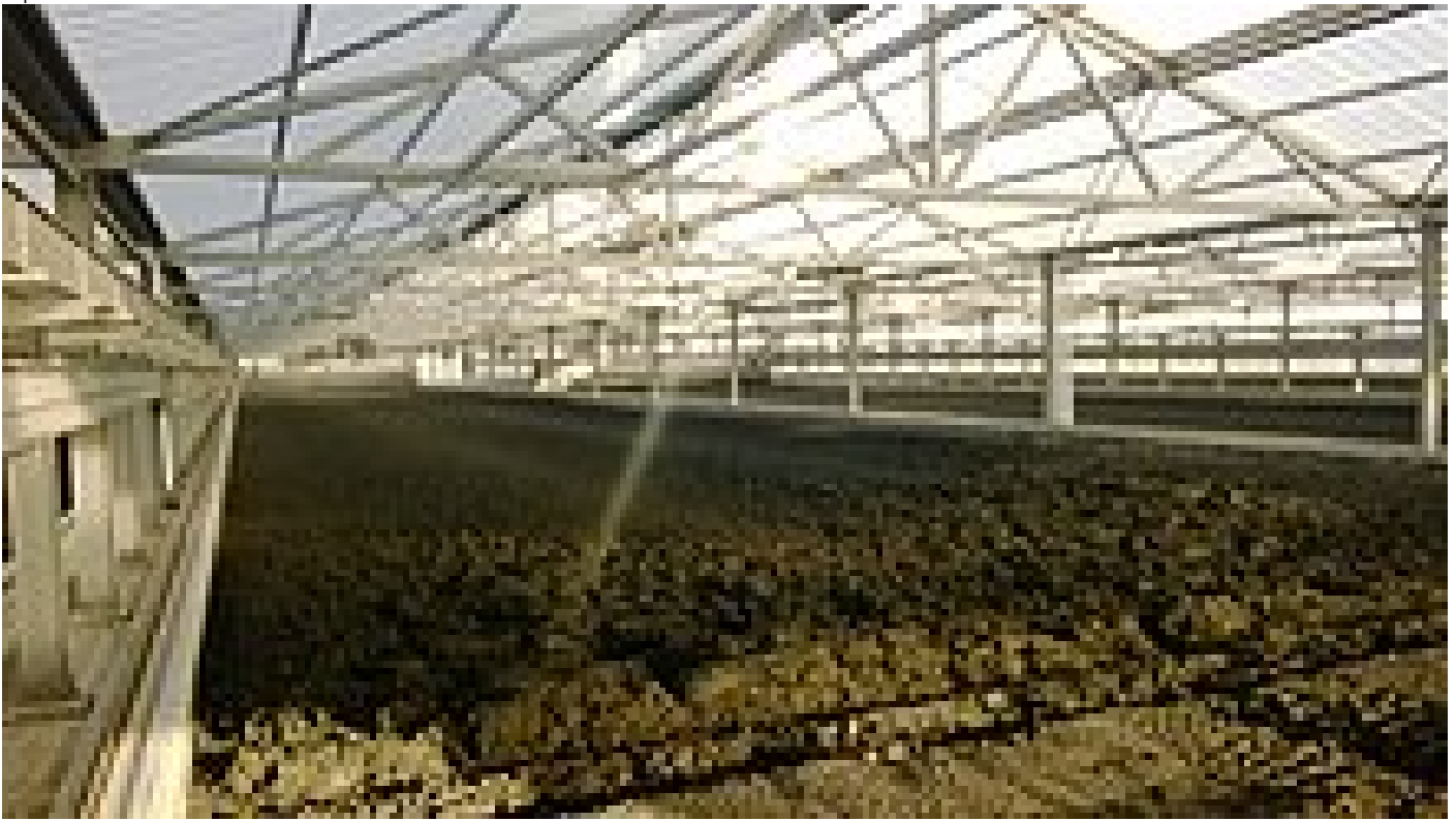
Eco-friendly reduction of disposal costs – sludge drying in a greenhouse
