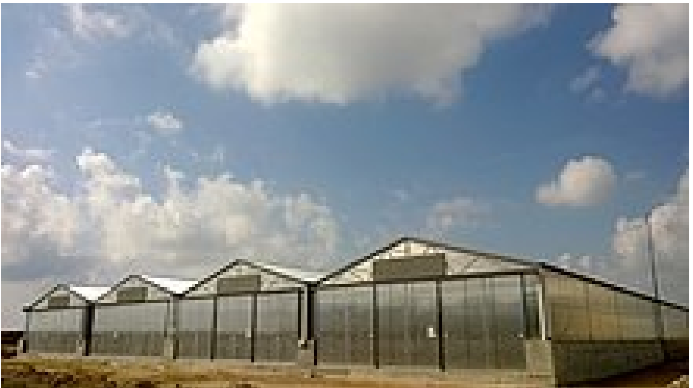
Increasing demand for large solar dryers – the method can reasonably be used also for huge sludge volumes
