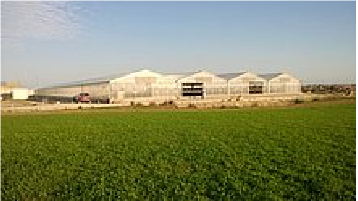
A place in the sun – sludge drying with simple means
