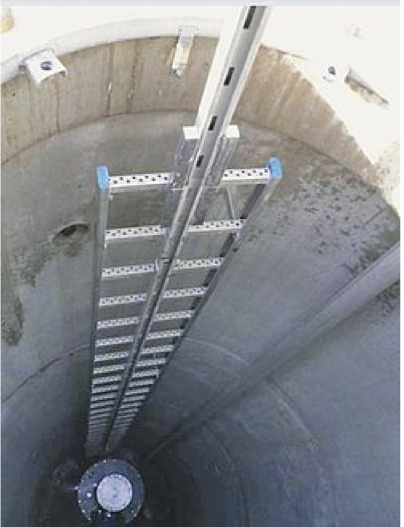
Safe access: ladder with safety guard rail
