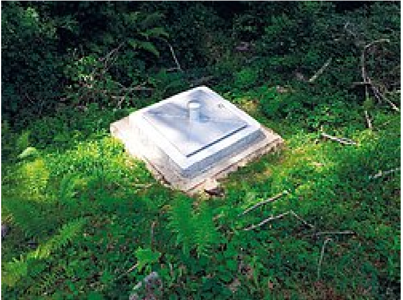
Shaft after refurbishment
