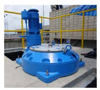
Reliable bull gear drive for the stirrer with airlift.
