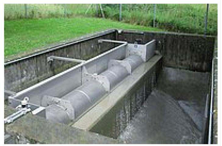
Automatically cleaned screen for solids retention in stormwater tanks and overflows
