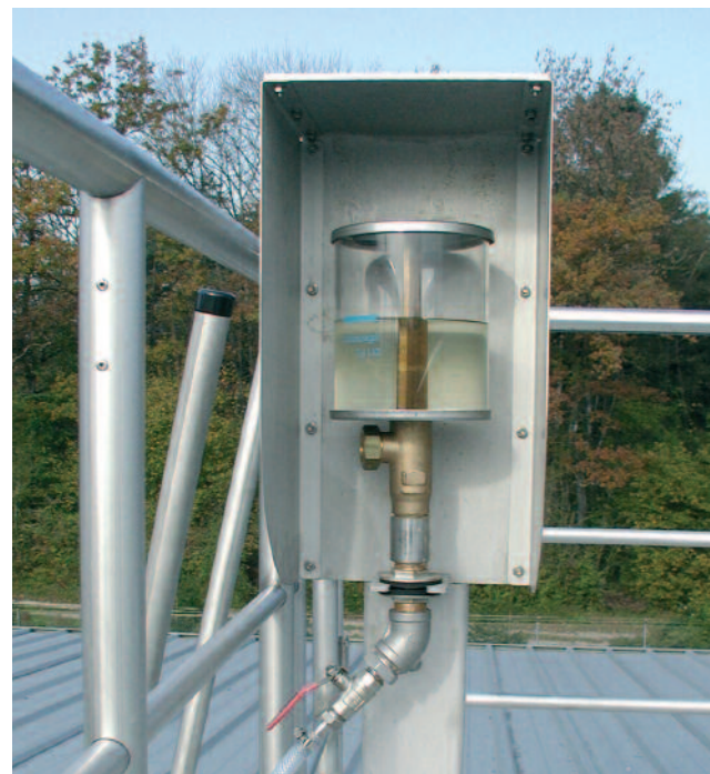
Leak control for VRM® bearing
