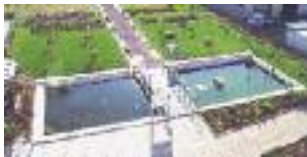
ReUse Park at HUBER Technology
