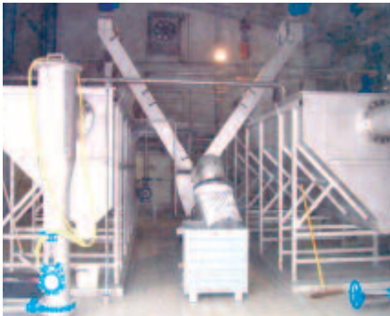
A pair of ROTAMAT® Complete Plants Ro5 discharging the screenings into a Washpress WAP
