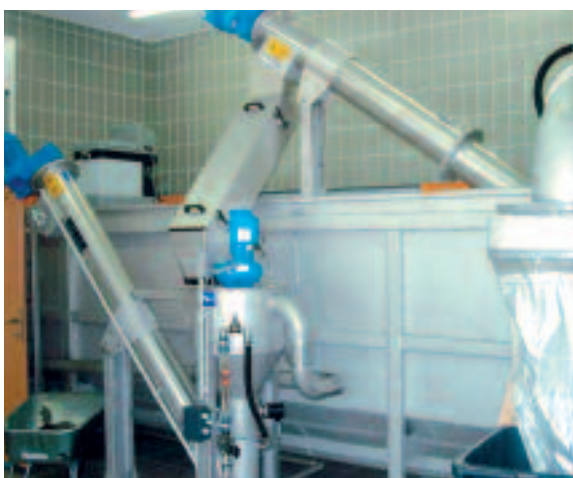
Classified grit slides from the inclined screw into a Grit Washer RoSF 4/t
