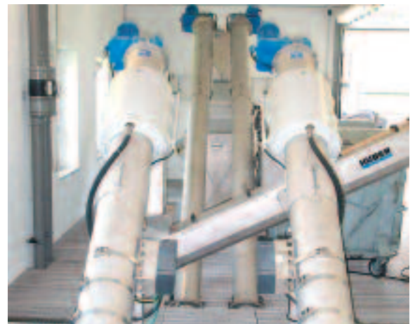
Below ground installation of a pair of Ro 5 Complete Plants
