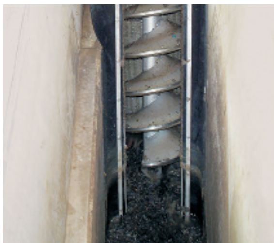
Extended version Ro 9 – XL; with shafted screw, maintenance-free bottom bearing and conical screw flights
