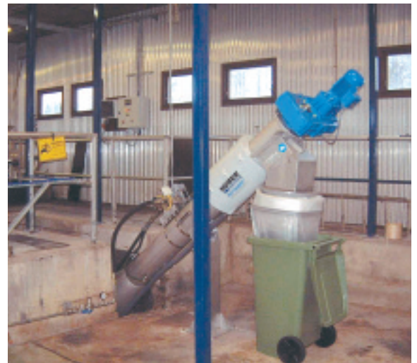
Indoor installation in a channel; with bagger
