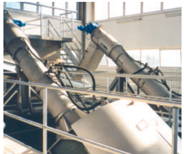
A pair of ROTAMAT® Fine Screens Ro1 with spray guards
